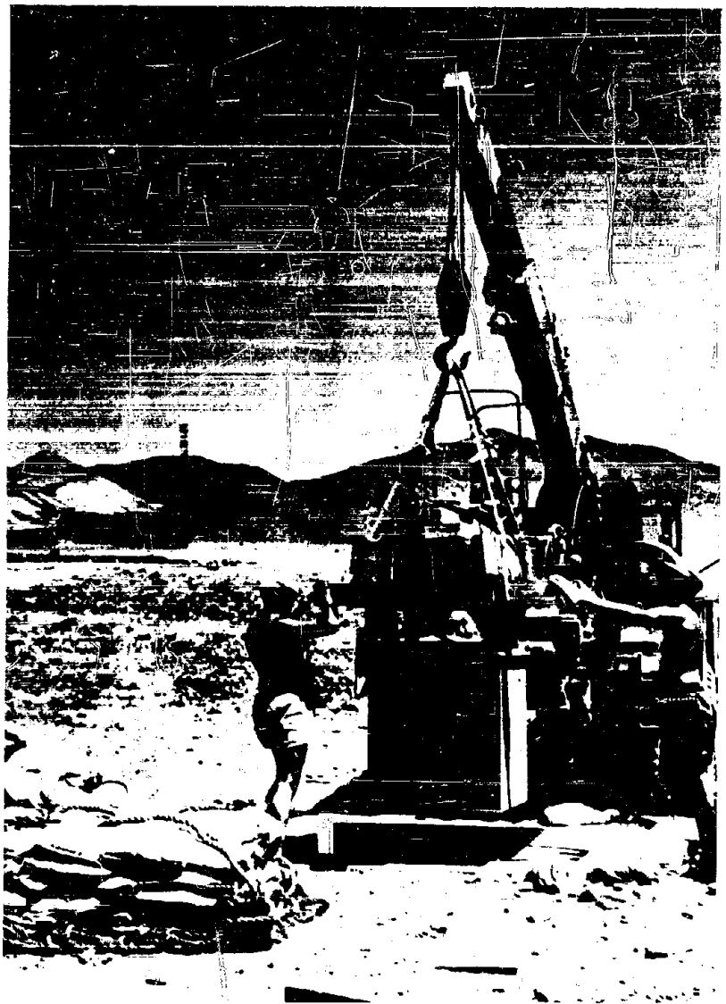
Figure 2.24 Lowering recording package into hole.
